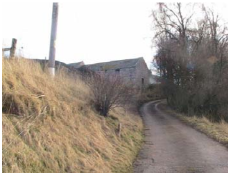
Fig. 2 : Existing watermill structure, as viewed from approaching access.
